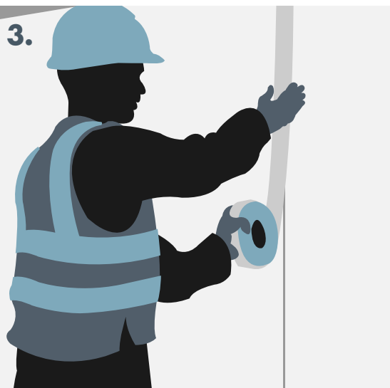
Taping the joints with Knauf Windliner Tape.
