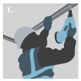
Fixing Knauf 'U' Channel – Perimeter Support to the soffit.
