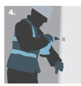
Fixing Knauf Plasterboard to the Knauf 'C' Channel.
