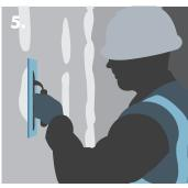
Applying Knauf Plasterboard Adhesive around the perimeter and at the required centres.
