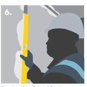
Ensuring Knauf Metal Furring Channels are fixed plumb.
