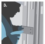
Bracing Knauf 'C' Studs with Knauf Fixing Channel at maximum 1500mm vertical centres (if required).
