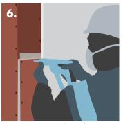
Fixing outer layer of Knauf Fire Panel.
