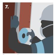
Taping and jointing encasement corners
