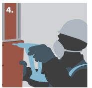
Fixing Knauf Fire Panel to Knauf 'C' Channels for horizontal joints.
