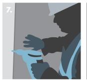
Fixing the 15mm Knauf Soundshield Plus to Knauf Acoustic 'C' Stud.
