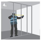
Twisting Knauf Acoustic 'C' Studs into position.
