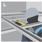
Measuring the distance between lower Knauf 'C' Channels.
