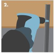
Fixing Knauf Angle Section as hanger.
