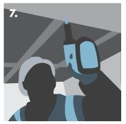
Screw fixing the Knauf Plasterboard to the lower Knauf 'C' Channels.
