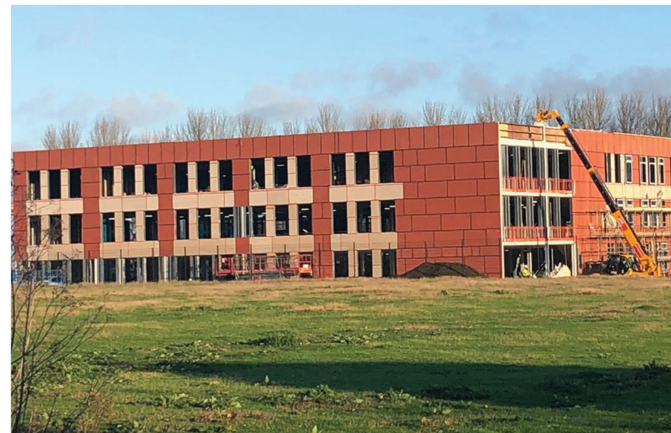
Knauf ThroughWall being installed at Leigh Academy Rainham, Kent
