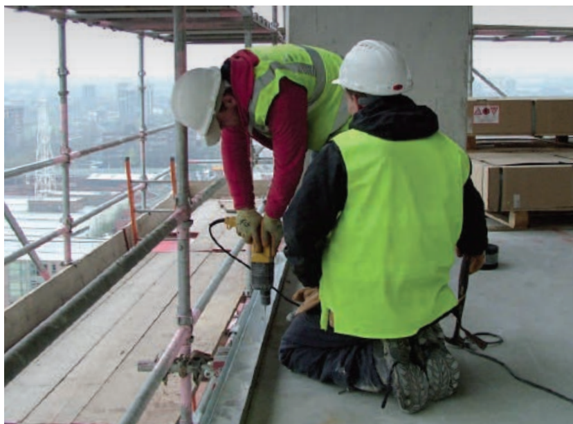
Figure 6.1 Fixing of base track to concrete slab
