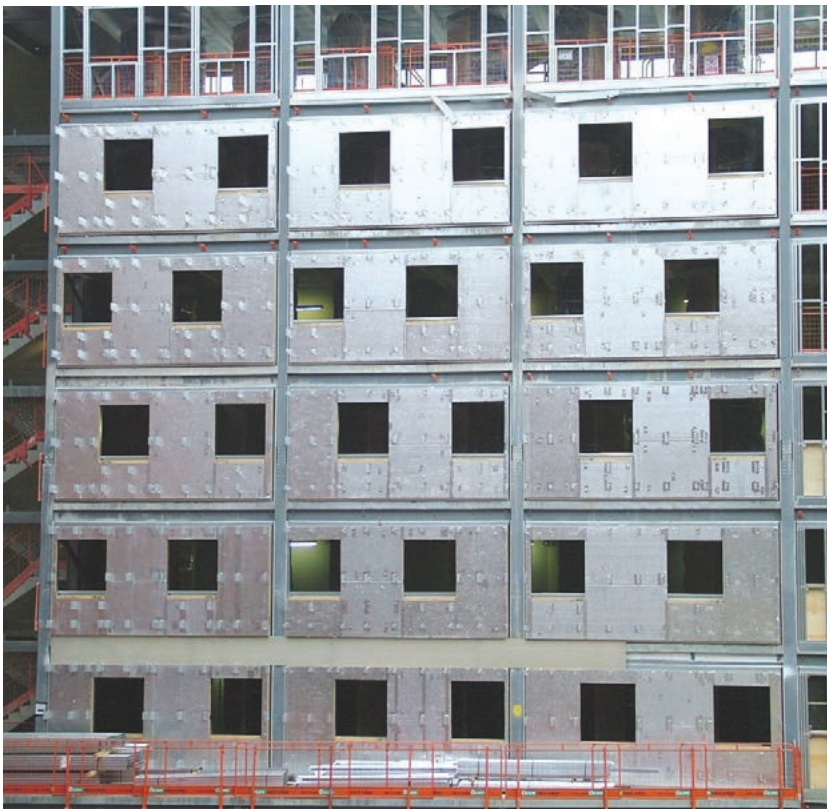
Figure 1.3 Typical prefabricated panelised external infill wall system
