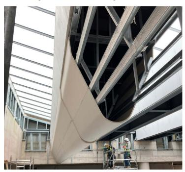
Knauf Curvex is a factory manufactured curved panel produced from 6mm thick gypsum board, and is used to form clean arcs or elliptical shapes.
