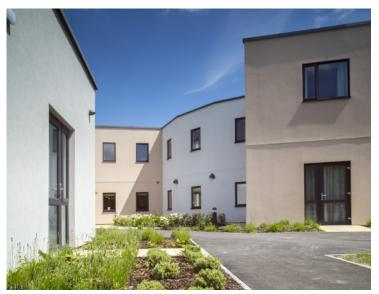
The decision to use Knauf AQUAPANEL® was made easier due to its characteristics as a directly applied render carrier board. The cement board combines the benefits of brick and block and, because it consists of aggregated Portland cement with coated glass fibre mesh embedded in the back and front surfaces, provides the ideal key for render.
