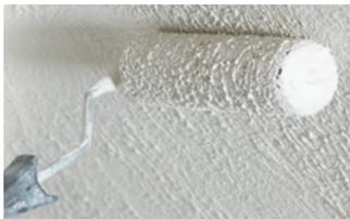
On textured backgrounds, apply Knauf ProRoll Max at a maximum of 2mm per coat, allowing each coat 12 - 18 hours to dry. Two coats of Knauf ProRoll Max can be applied if required, followed by a 1mm coat of Knauf ProRoll Light to finish. On smooth backgrounds, just Knauf ProRoll Light is required in coats of 1mm up to a maximum of 3mm.
