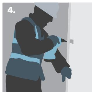
4. Fixing Knauf Plasterboard to the Knauf 'C' Channel.
