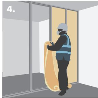
4. Inserting Knauf insulation quilt between the Knauf 'C' or 'I' Studs.
