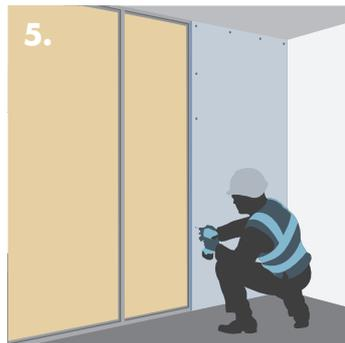
5. Fixing Knauf Plasterboard to the Knauf 'C' or 'I' Studs.
