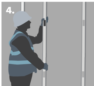
4. Adjusting the stud position.
