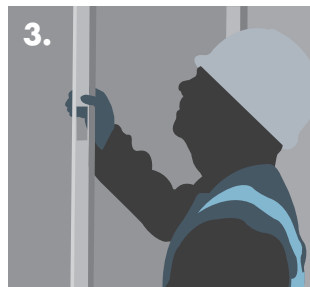
3. Twisting Knauf 'I' Studs into place.
