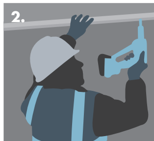
2. Installing head track.
