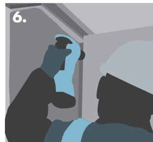
6. Fixing Knauf Plasterboards to complete the lining.
