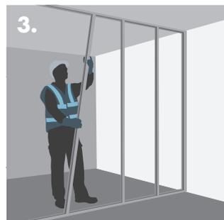
3. Twisting Knauf Acoustic 'C' Studs into position.
