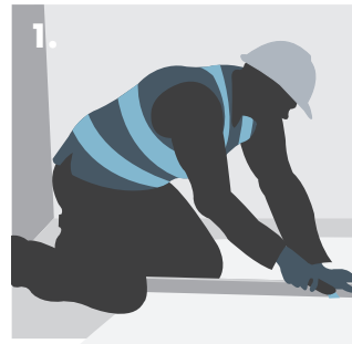
1. Scoring Knauf Aquapanel Exterior with a knife.
