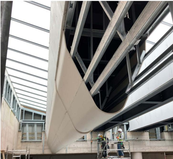
**Knauf Curvex is a factory manufactured curved panel produced from 6mm thick gypsum board, and is used to form clean arcs or elliptical shapes.**
