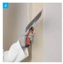
Apply second coat to 175mm each side of the corner.
