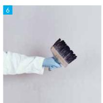
Applying Knauf Wallboard Primer for Tape & Jointing system only.
