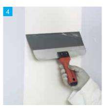
Applying the second coat of Knauf Joint Cement Premium.
