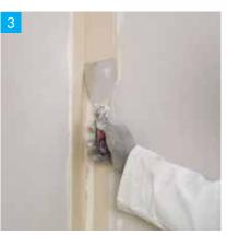
Cover to a width of 50mm each side of the joint.
