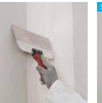
Apply Knauf Joint Cement Premium finish coat to 75mm each side.
