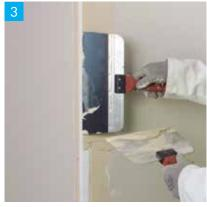
Applying the first layer of Knauf Joint Filler Premium.
