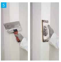
Applying the finish coat of Knauf Joint Cement Premium.
