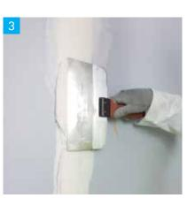
Applying first coat of Knauf Joint Cement Premium.
